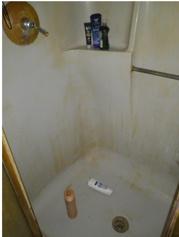
Second floor shower
